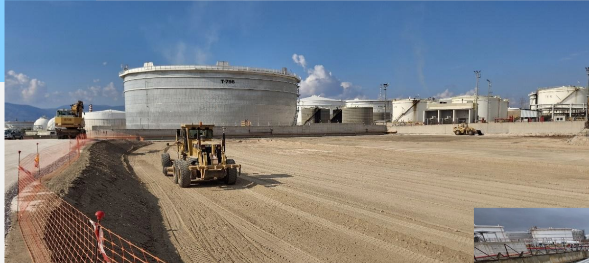
Earthworks for Electrolysis Unit
